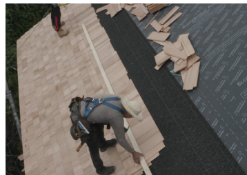
Cedar Shingles/Shakes With VaproMat™ Drainage Matrix
